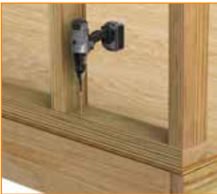
BOTTOM PLATE TO RIM BOARD
